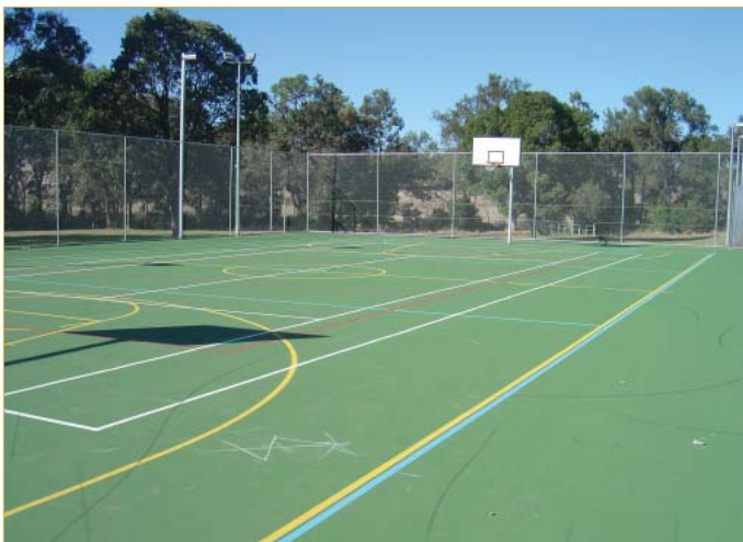
Multi-purpose court at Errol Munt Sports Centre - Yarraman
