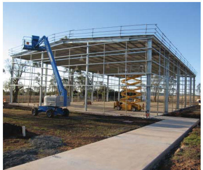
Bunkers Hill State School indoor hall under construction
