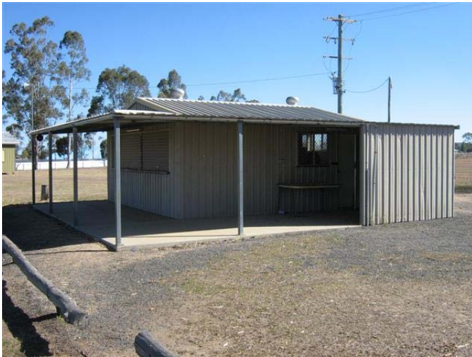
Metal framed metal clad structure with metal roof.
