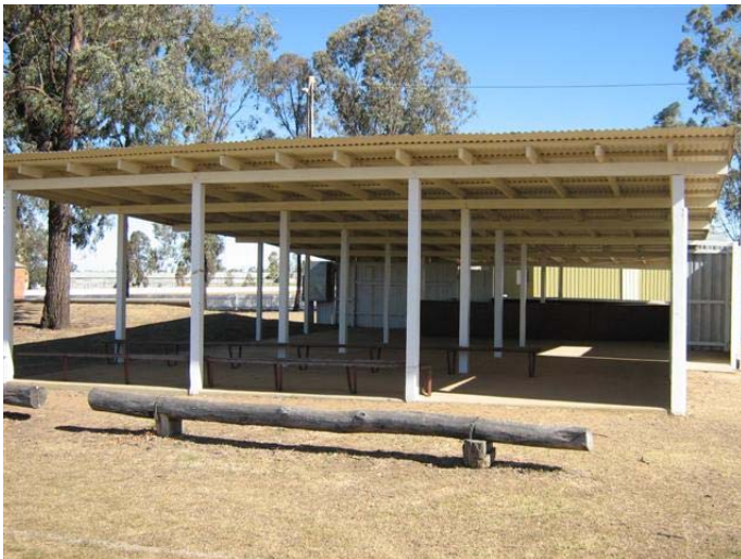
Timber framed structure, timber/metal clad, with metal roof. No services.
