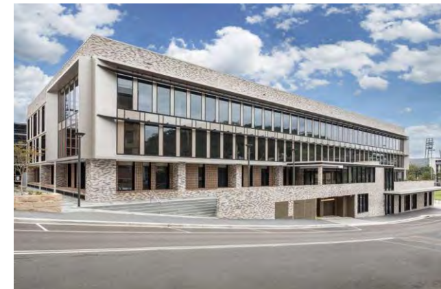
New ATO building. Source: domagroup.com.au
