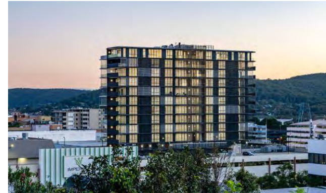
Bonython Tower. Source: Stevens Construction
